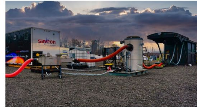
Phase 3: Pilot Scale Tests Field Implementation
