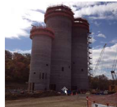
Slip Form Construction for Fly Ash Silos
